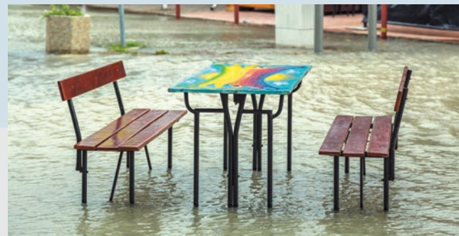
D No Drainage
